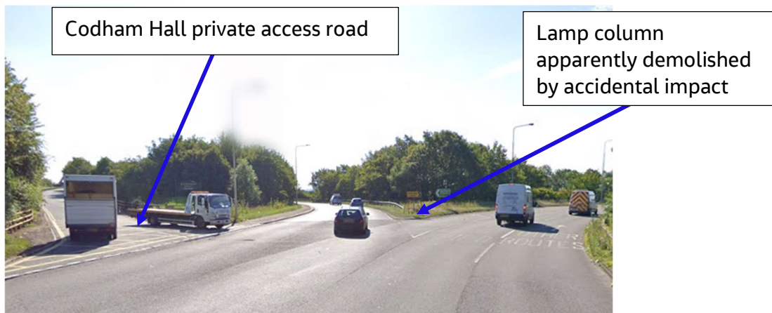
FIGURE 3-31 – GOOGLE STREETVIEW IMAGE OF CODHAM HALL ENTRY
